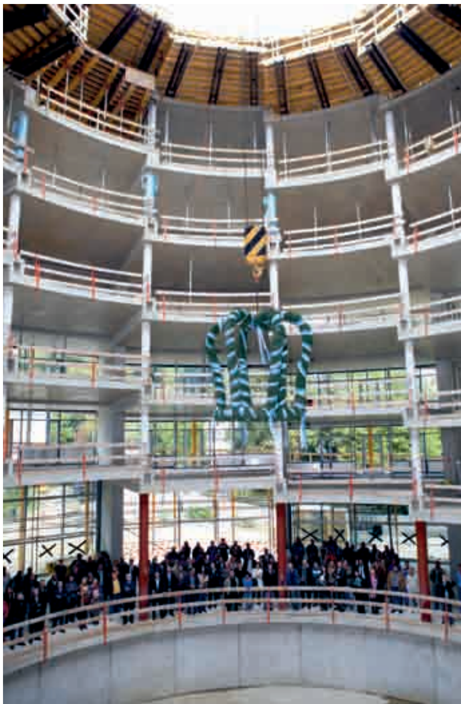
ATC topping out ceremony
