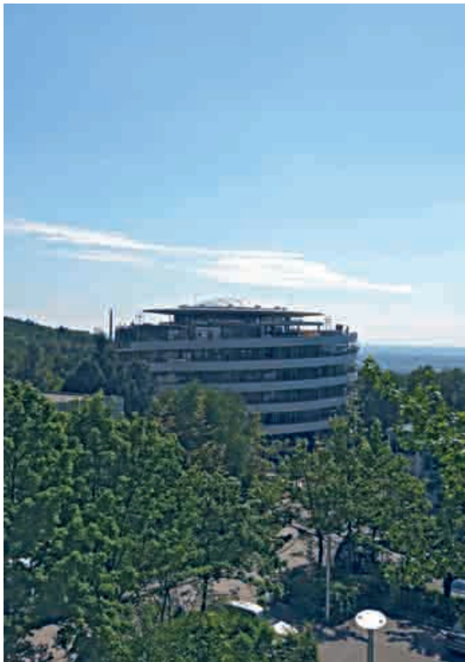
The Advanced Training Centre on the Heidelberg campus is close to completion.
